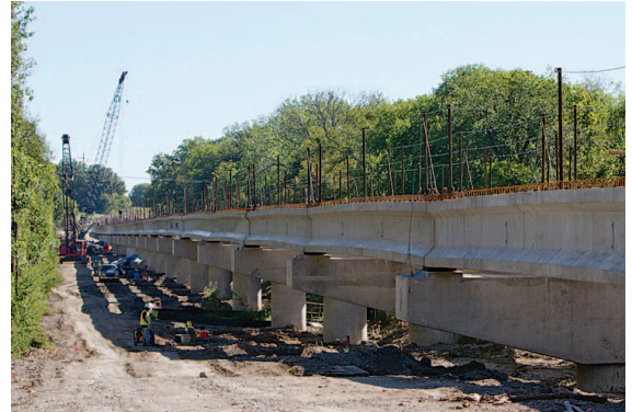
Rowlett Creek Light Rail Bridge
